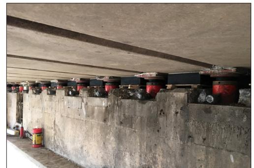
*Bespoke, low-height abutment jacking accommodates the structure's height restriction between bridge pier and soffit*
