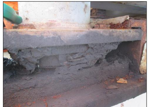
*Existing bearing prior to removal shows excessive corrosion*
