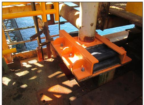
*Bearing replaced complete with protective cover*
