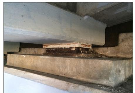
*Old rocker bearing corroded and no longer functional*
