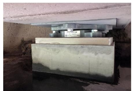
*New installed mechanical pot bearing fixed to the bridge beam and bearing shelf*
