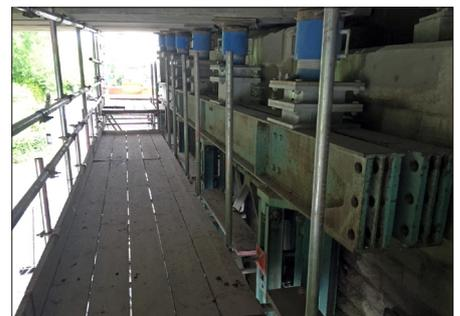
*Super props and jacks temporarily supporting the bridge deck*
